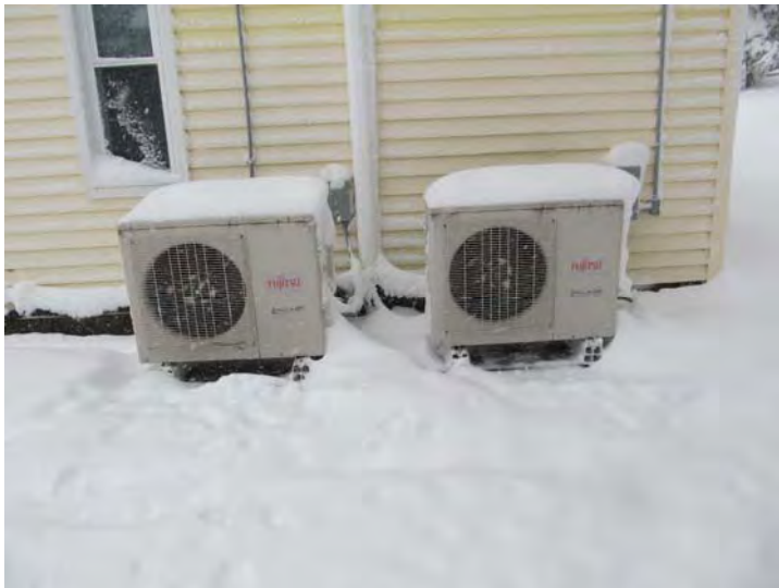
Exterior condensers for recently installed heat pump systems serving each apartment
