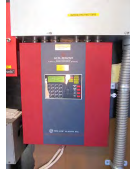
Common area and in-unit smoke/fire detection devices monitored by a contemporary fully addressable fire alarm control panel
