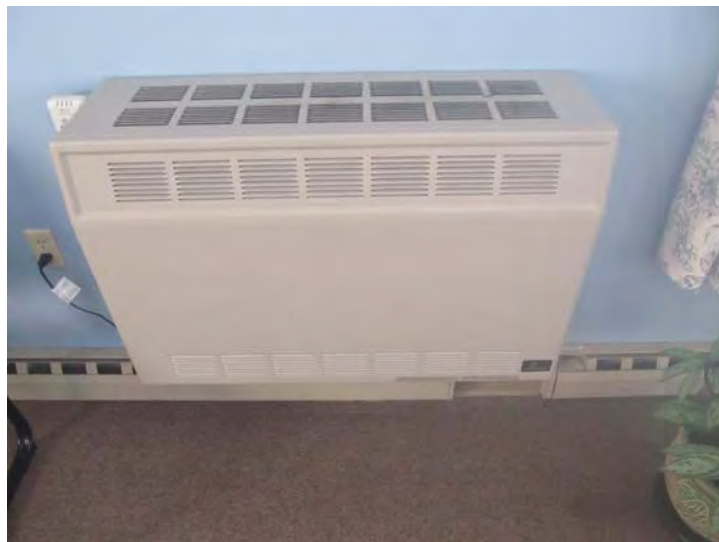
Propane-fired wall furnace serving community room
